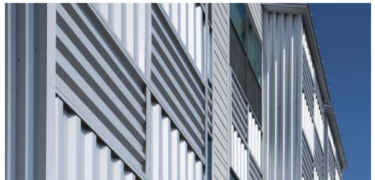
Pictured Above Project: NOBAY Village Architect: WMB-ROI Architecture General Contractor: RODDA Construction, Inc. Installing Contractor: CA Systems Color: Acrylic-Coated Galvalume®
